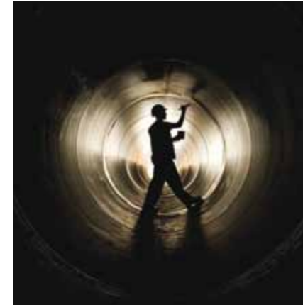
The new pipe bridge will help to improve water quality in the River Calder
